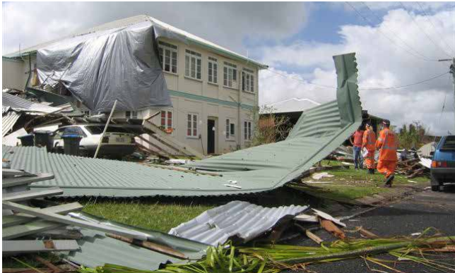
Figure 32: Damage to buildings in Yeppoon in the aftermath of Cyclone Marcia, 2015. Source: Queensland Fire and Emergency Services
