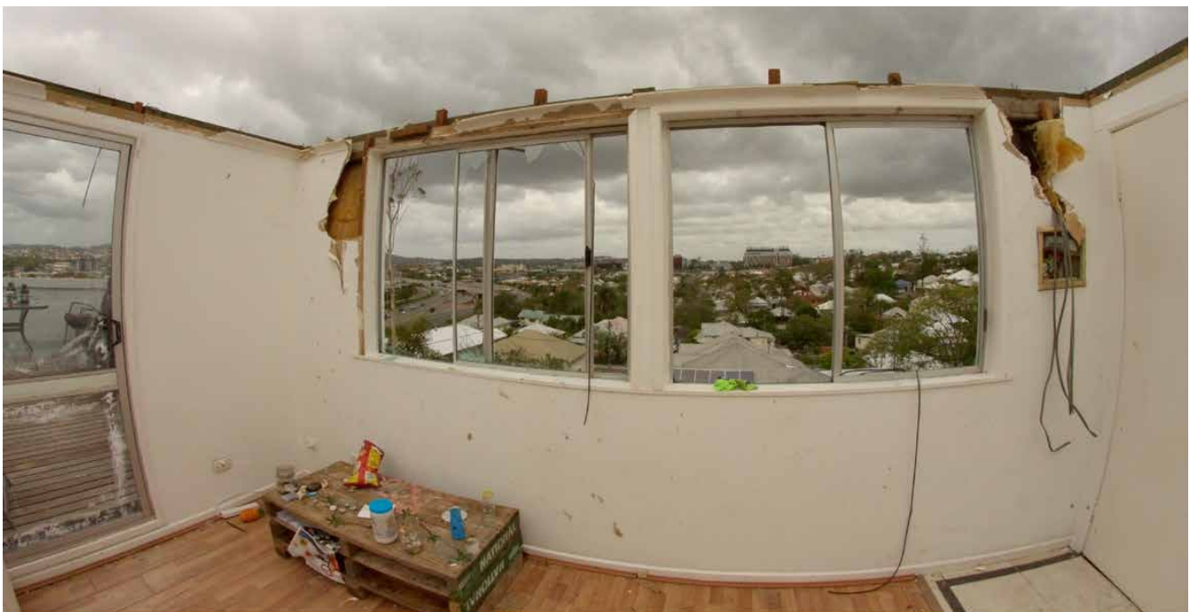
Figure 67: A super cell hit Brisbane on November 28, 2014, causing widespread destruction in a short period of time. In this photo, a roof has been removed from a block of flats. Source: paintings/Shutterstock.
