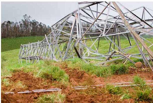
Figure 47: Fallen transmission lines as a result of Cyclone Yasi, 2011. Source: Powerlink
