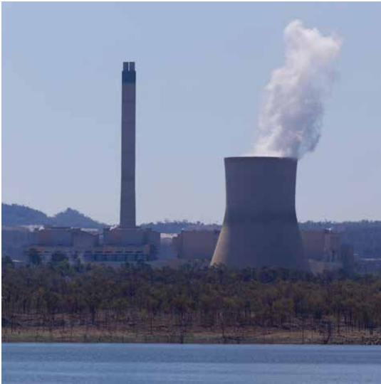
Figure 105: Callide coal fired power station. Source: Alamy
