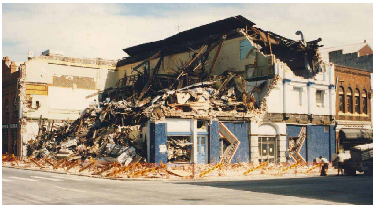
Figure 86: Damaged caused by the 1989 Newcastle earthquake was significant and destructive. In this photo, the RSL club is almost completely destroyed. Source: Telstra Museum, Newcastle
