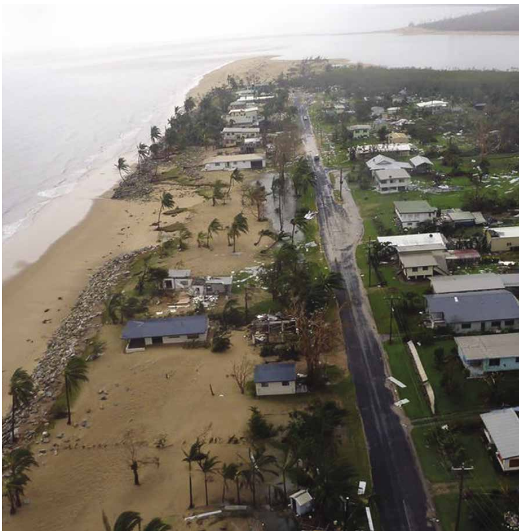
Figure 22: The effects of storm surge at Tully Heads from Tropical Cyclone Yasi in February 2011. Source: ABC News (Kerrin Binnie)
