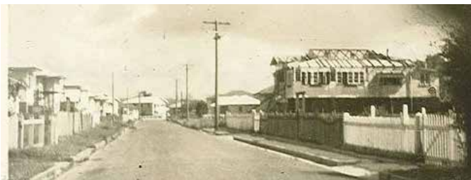
Figure 26: Roof Loss in Norman Street, 1954 Great Gold Coast Cyclone.
