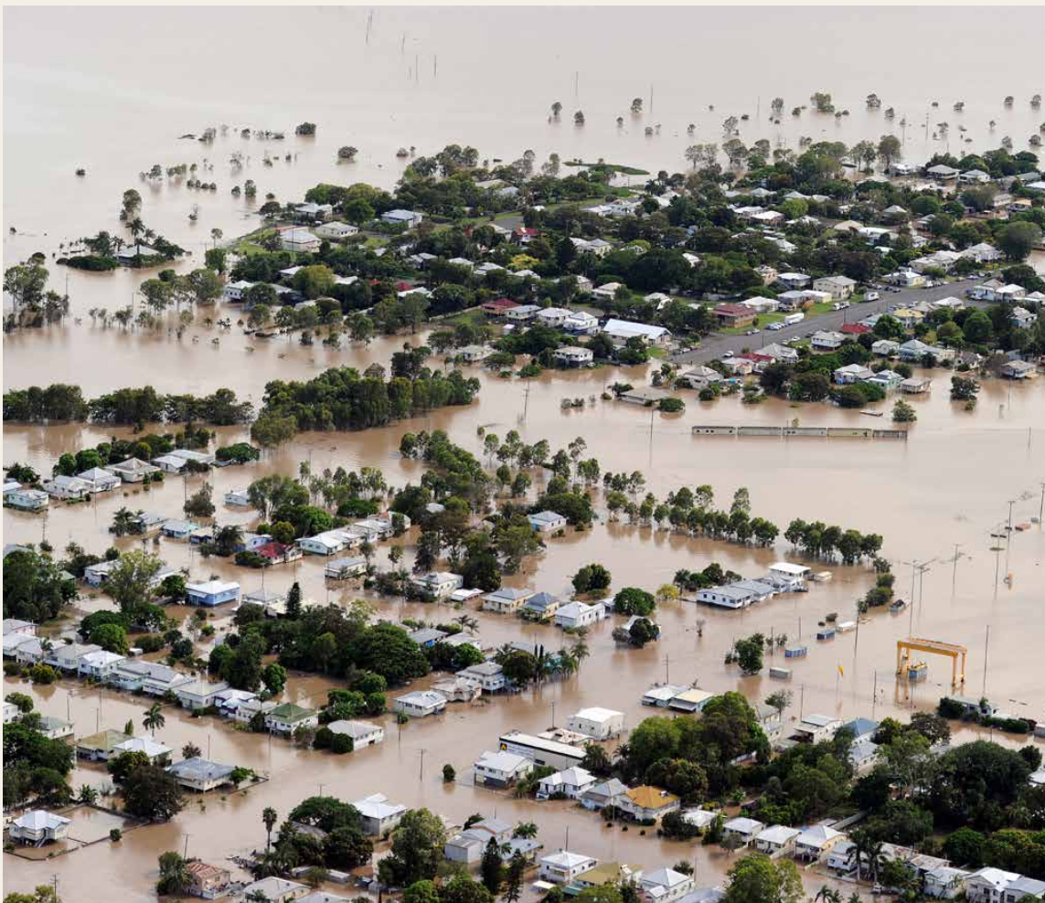
Figure 63: Bundaberg flood, 2013. Source: Image courtesy of Torsten Blackwood.
