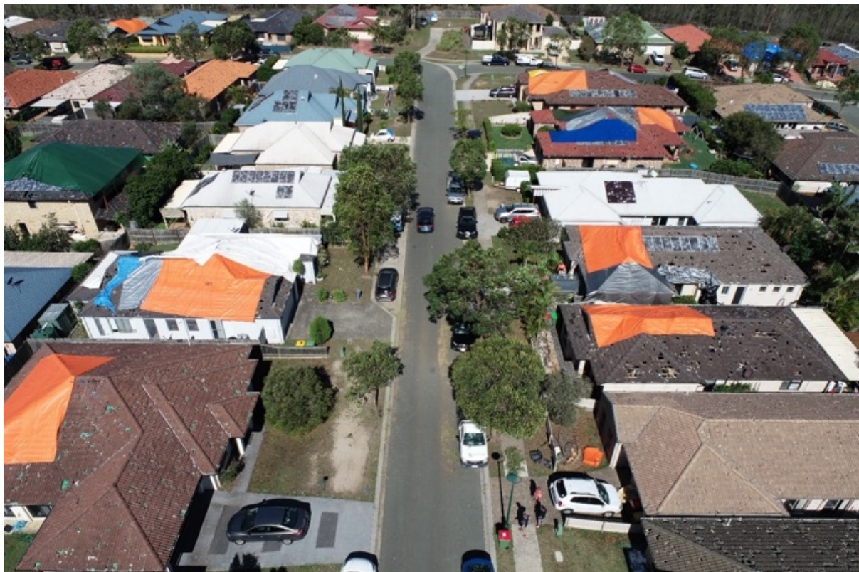
Figure 69: Extensive hail damage following the severe thunderstorms that impacted South-East Queensland on 31 October, 2020. Source: QFES.
