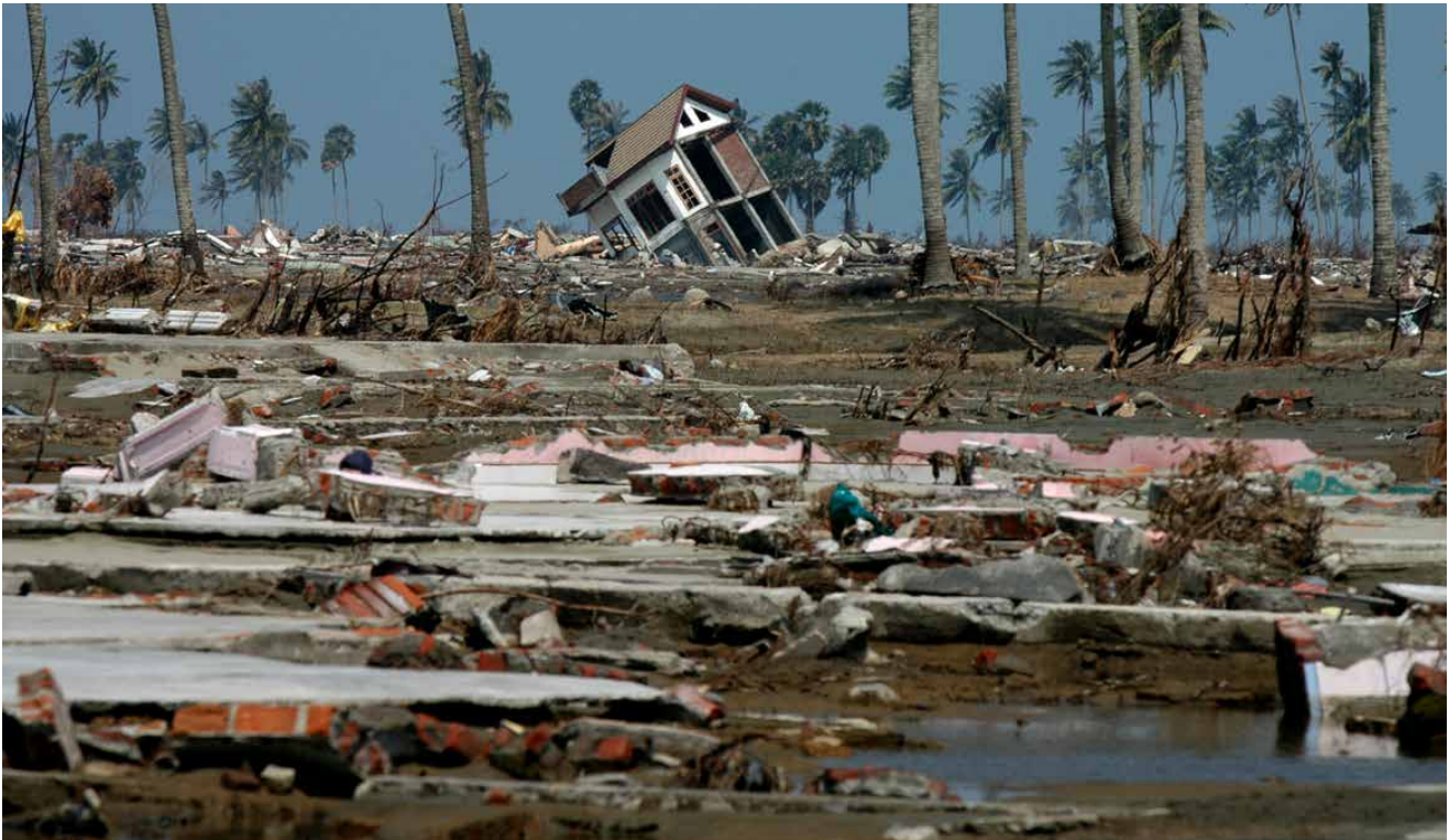
Figure 93: Impacts of the 26 December, 2004 Indian Ocean earthquake and tsunami in Banda Aceh City, Indonesia. Hundreds of thousands of people lost their lives as a result of the earthquake and associated tsunami. Source: Shutterstock.
