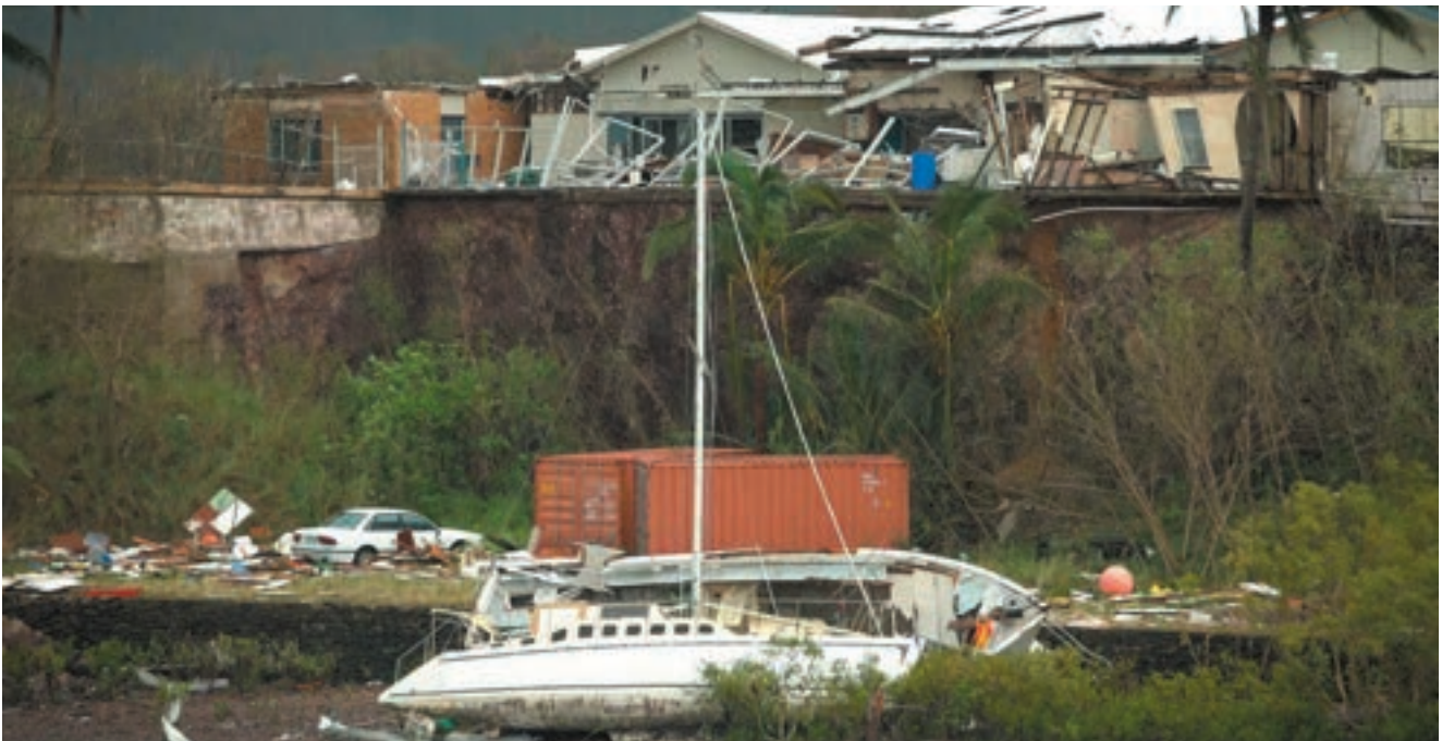
Figure 53: Shute Harbour is littered with debris following Cyclone Debbie. Source: AAP (Dan Peled)
