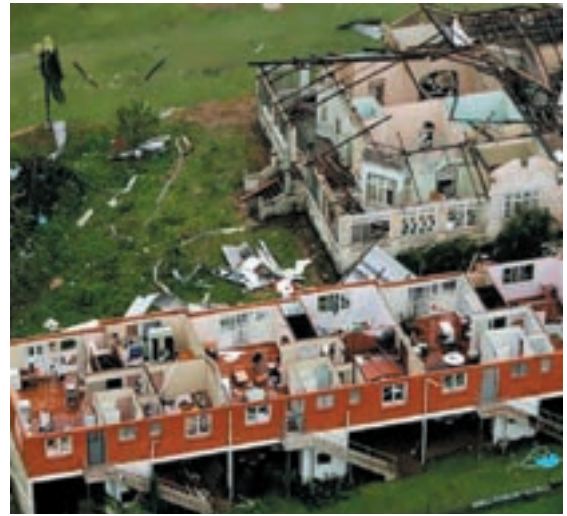
Figure 88: Houses and apartment blocks with their roofs blown off in Innisfail after Cyclone Larry struck in March 2006. Source: AP (Mark Baker)
