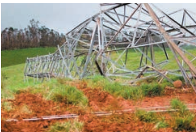
Figure 112: Fallen transmission lines as a result of Tropical Cyclone Yasi, 2011. Source: Powerlink
