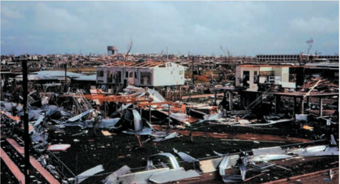
Figure 121: The suburb of Alawa, after Cyclone Tracy hit - Christmas Day 1974
