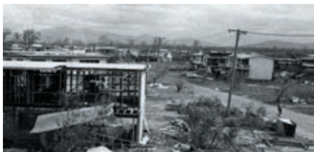
Figure 64: The suburb of Pallarenda, after Cyclone Althea in December 1971. Source: CityLibraries Townsville Local History Collection
