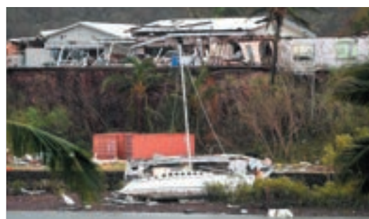
Figure 2: Damage to Shute Harbour. Source: ABC News (Dan Peled)
