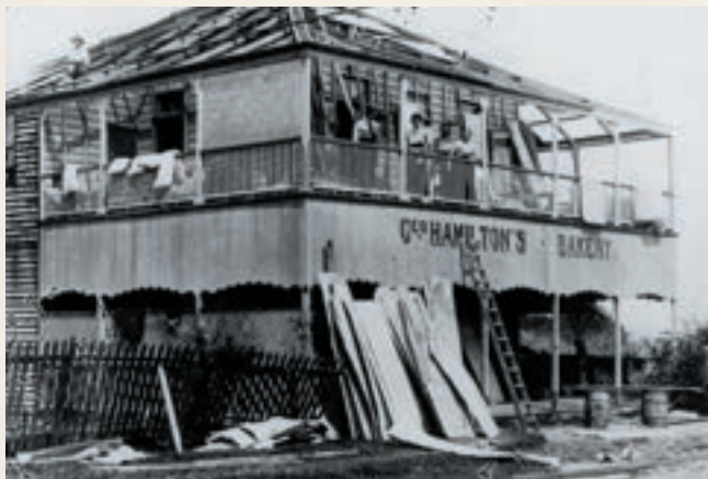
George Hamilton's Bakery damaged post impact.
