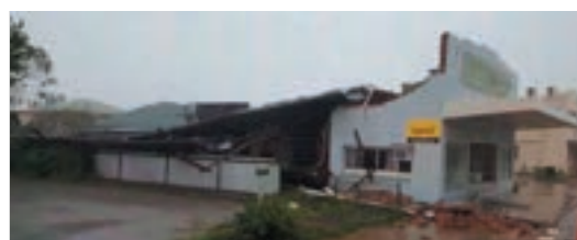
Figure 3: A badly-damaged plumbing business in Proserpine, 101km north west of Mackay. Source: ABC News
