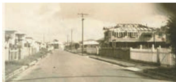
Figure 25: Roof Loss in Norman Street
