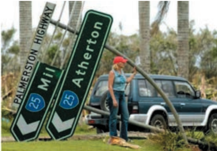
Figure 85: A road sign bent by the wind in Innisfail after Cyclone Larry in March 2006. Source: ABC
