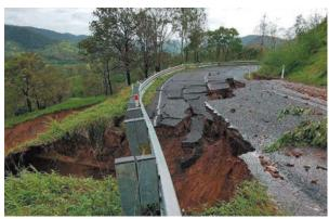
Figure 26: Serious damage around Sarina Range due to landslips from Severe TC Debbie. Source: Loretta MacGregor
