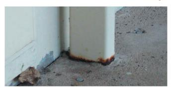
Figure 12: Signs of rust at the bottom of a verandah post.
