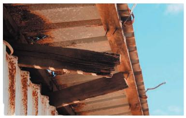
Figure 13: Timber rot in a rafter.
