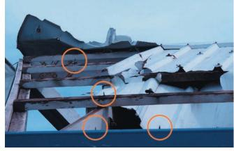
Figure 11: Roof failure occurred due to corroded roofing fasteners.
