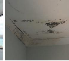
Damage to plasterboard ceiling from water ingress through the roof.
