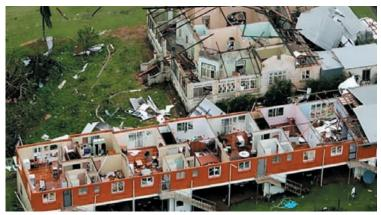
Figure 21: Houses and apartment blocks with their roofs blown off in Innisfail after Severe TC Larry struck in March 2006. Source: Mark Baker(AP)
