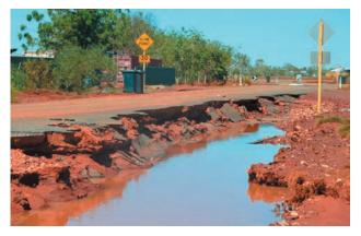
Figure 10: Scour damage to a road from storm surge.
