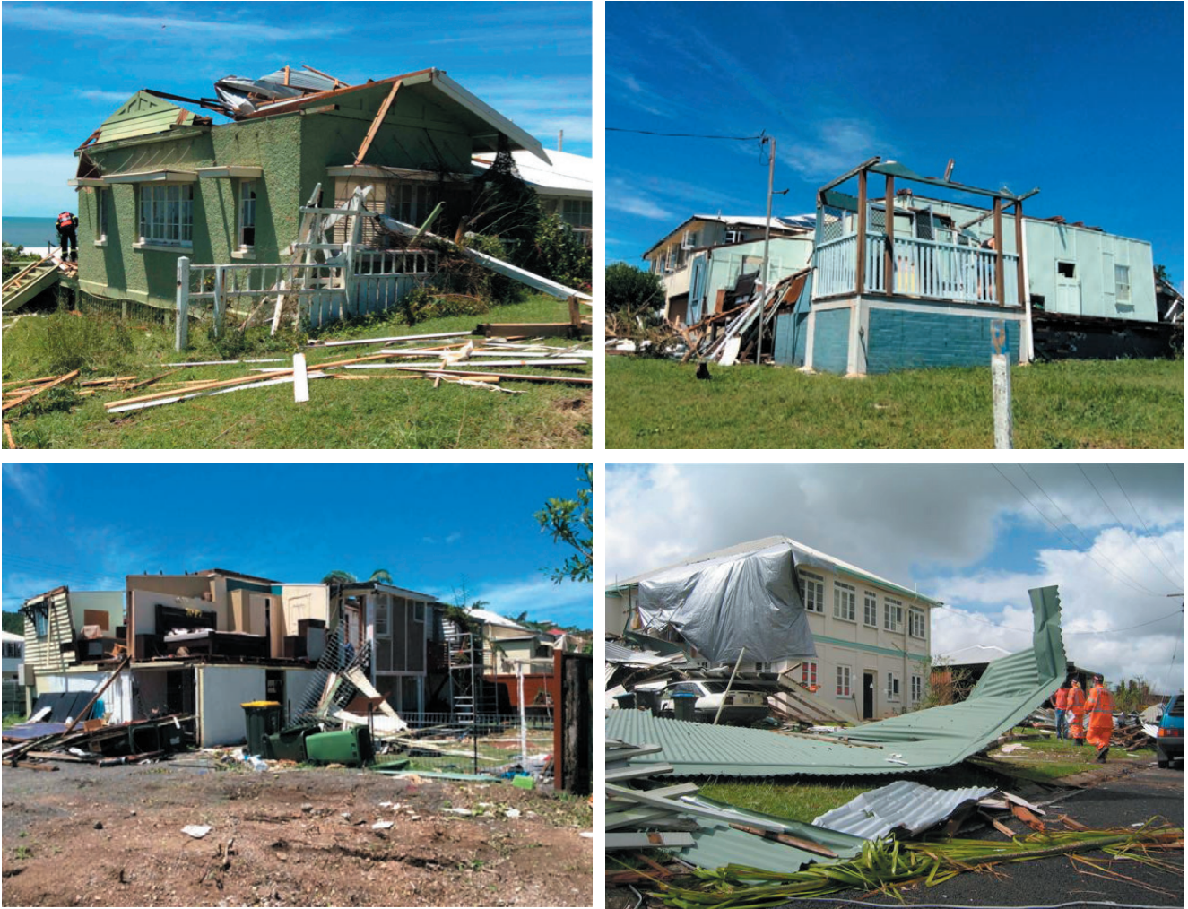
Figure 2: Damage to buildings in Yeppoon in the aftermath of Tropical Cyclone Marcia, 2015. Source: QFES
