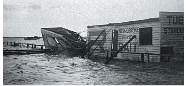
Figure 10: Storm surge at Tuesleys Jetty, Southport - 1954 Great Gold Coast Cyclone.
