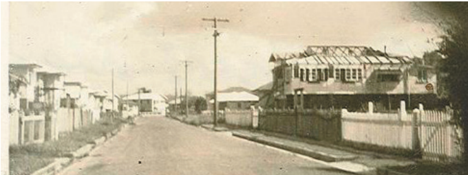
Figure 11: Roof Loss in Norman Street, 1954 Great Gold Coast Cyclone.
